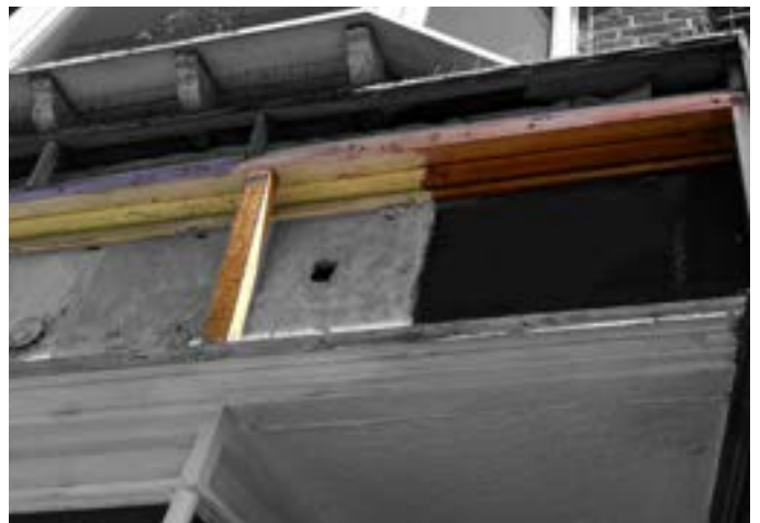
An example of an additional horizontal, timber batten supported by vertical post and used to achieve an angled fascia.
