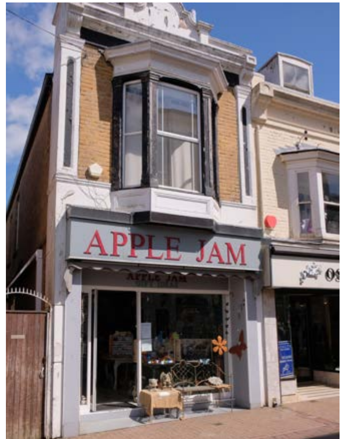
The engaged pilasters on this shop's upper storey would once have framed the entire façade
