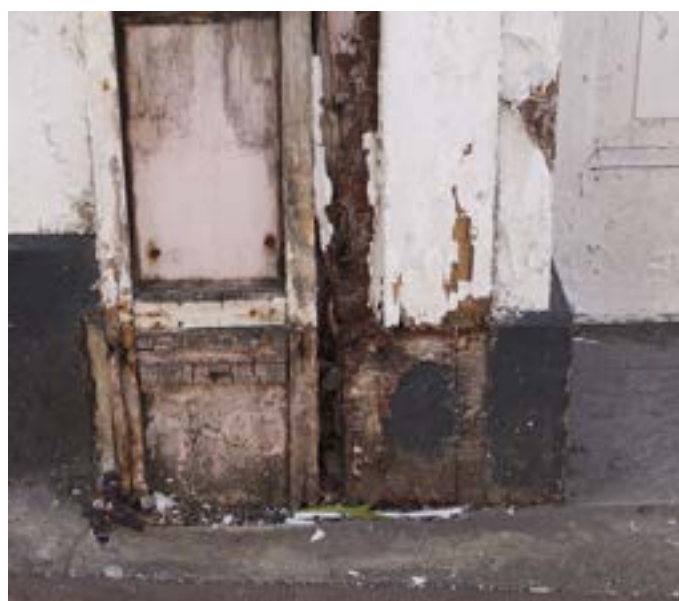
Timber stallriser suffering from bad damp
