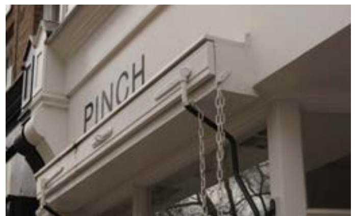
A well fitted, non-integrated shop blind, London
